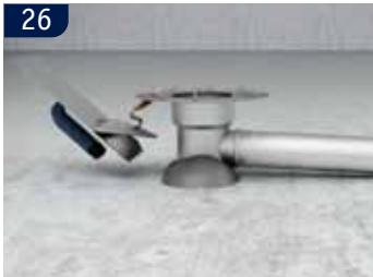
**UK** To make sure that the drain will not float upwards during casting, it is recommended that the drain lower part is haunched in concrete.
