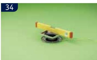
**UK** Adjust the upper part to the correct height and make sure it is level. BLÜCHER recommends using the 4 adjustment screws to ensure that the upper part is 100% level.
