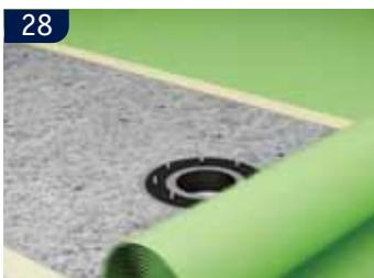
**UK** Install the (flat) sealing ring
