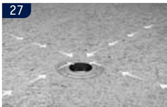
**UK** Cast the floor with the recommended fall towards the drain.
