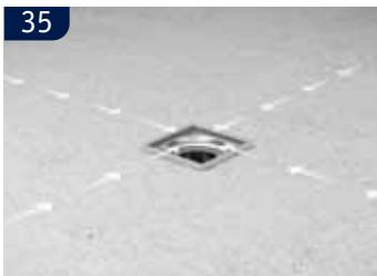
**UK** Cast the floor with the recommended fall towards the drain. Lay the tiles.
