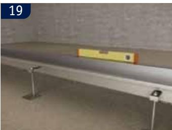
**UK** Adjust the height of the channel to the correct height and make sure it is level. BLÜCHER recommends using adjustable legs type 670.000.00X (to be ordered separately)
