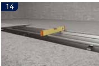
**UK** Adjust the channel to make sure it is level and in the correct height for the finished tiled or resin floor height. Partially infill the void with concrete
