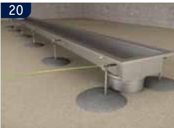
**UK** To make sure that the channel will not float up during casting, it is recommended that the feet of the adjustable legs are set in concrete. If an equipotential bonding is required, connect the earth wire to one of the adjustable legs.
