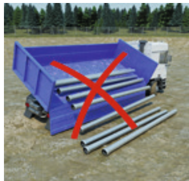
Pipes and fittings must not be dumped off trucks.
