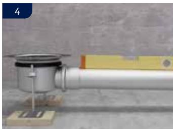
**UK** Connect the outlet to the drainage pipe. Establish correct fall of the drainage pipe.
