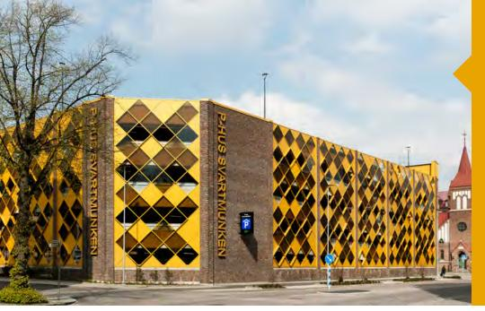
The parking garage Svartmunken was built in the city center of Halmstad in Sweden with a modern design and with five different floors accommodating a total of 360 parking spaces on an area covering 9400 m². On the bottom floor the floor type is draining asphalt and on the other floors it is asphalt concrete.
